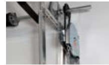
Hand chain hoist with an integral braking system provides controlled descent for sectional doors.
